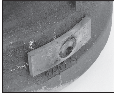
Welded balance weight
